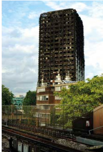
ABOVE: The remains of Grenfell Tower following the devastating fire in 2017
